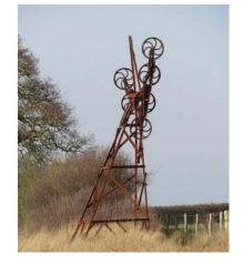
Ballast Barge Jetty in Alresford Creek and the three Bucket Chain Pylons leading to it are monuments of ongoing gravel works from a time when bulk loads going a distance were carried by barge. This was probably why it was necessary to have a swing bridge across the creek for the now closed Wivenhoe to Brightlingsea railway.
